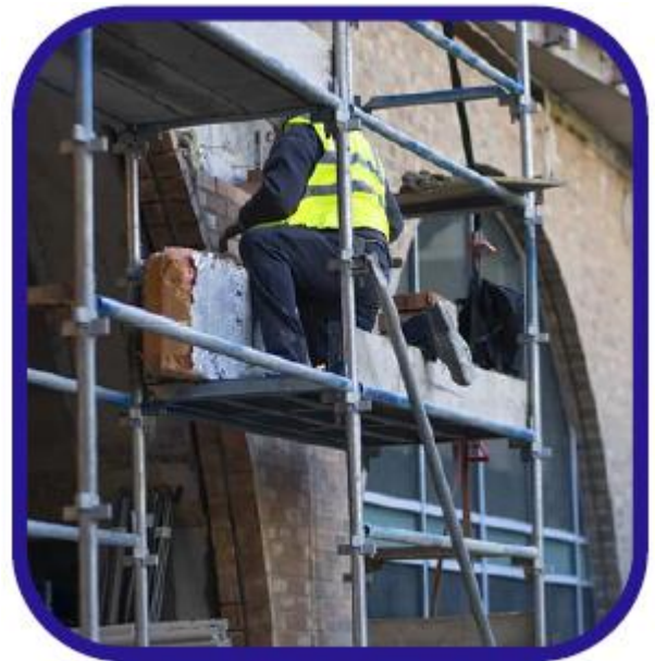
MALING SCAFFOLDING WORK
